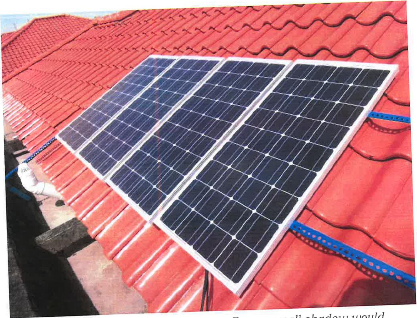
*Figure 1: A typical domestic solar array. Even a small shadow would result in the power output being reduced from the affected panels.*
