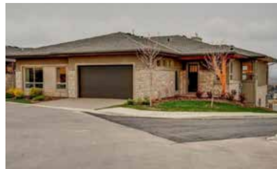
The built environment will be designed to be compatible with the natural environment.
