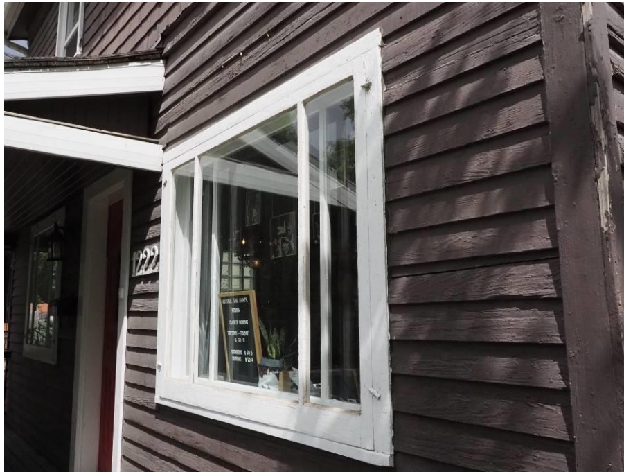
(Image 2.7 – Window detail on south façade with storm sash)
