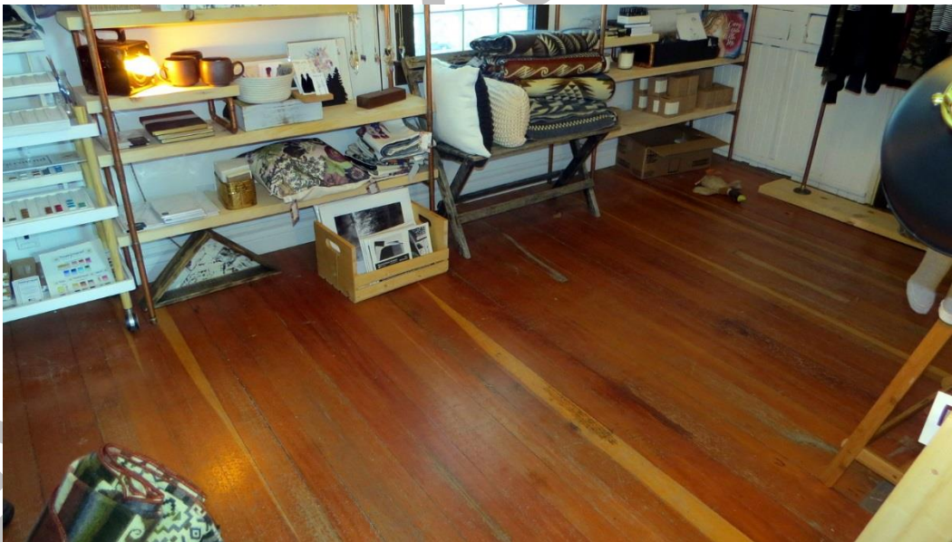
(Image 3.4 – Detail of wood flooring on first storey)
