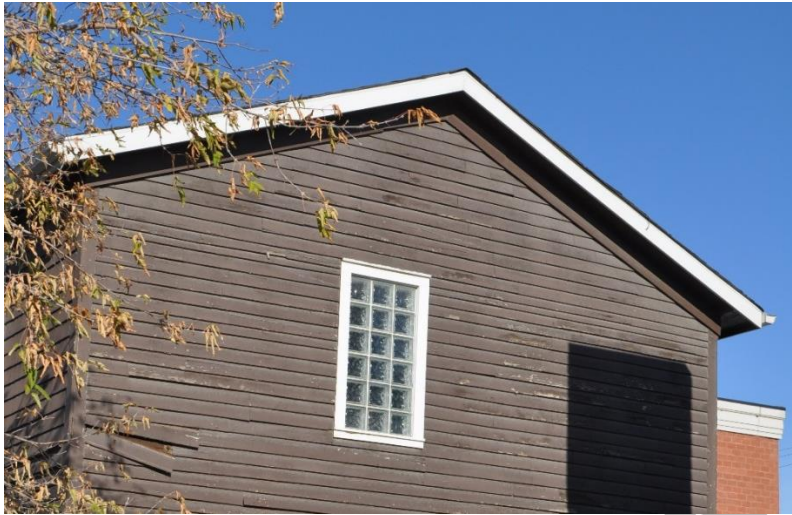
(Image 2.9 – West façade showing verge boards)
