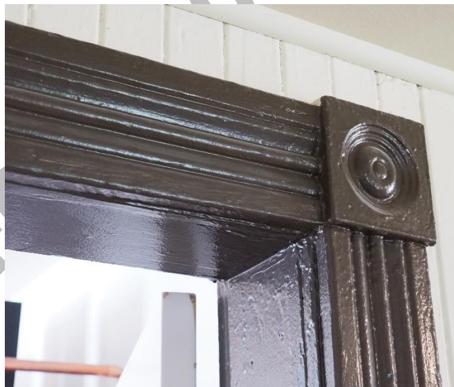
(Image 3.6 – Detail showing example of historic door surround)
