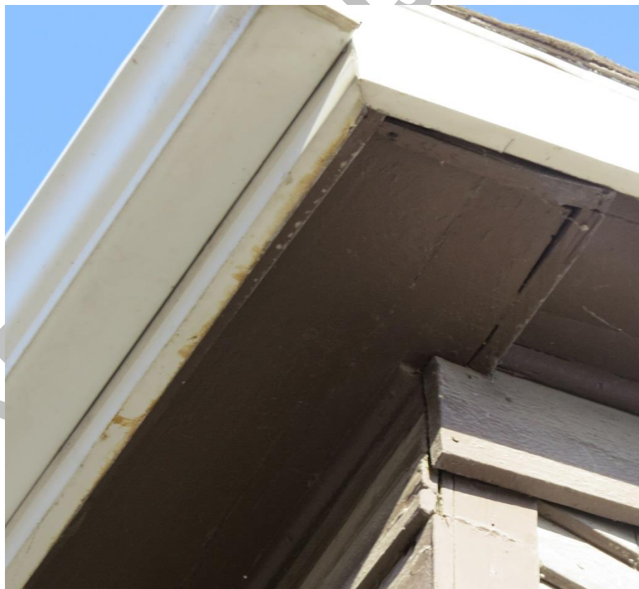
(Image 2.8 – Detail of wood soffits, fascia, verge boards and frieze)
