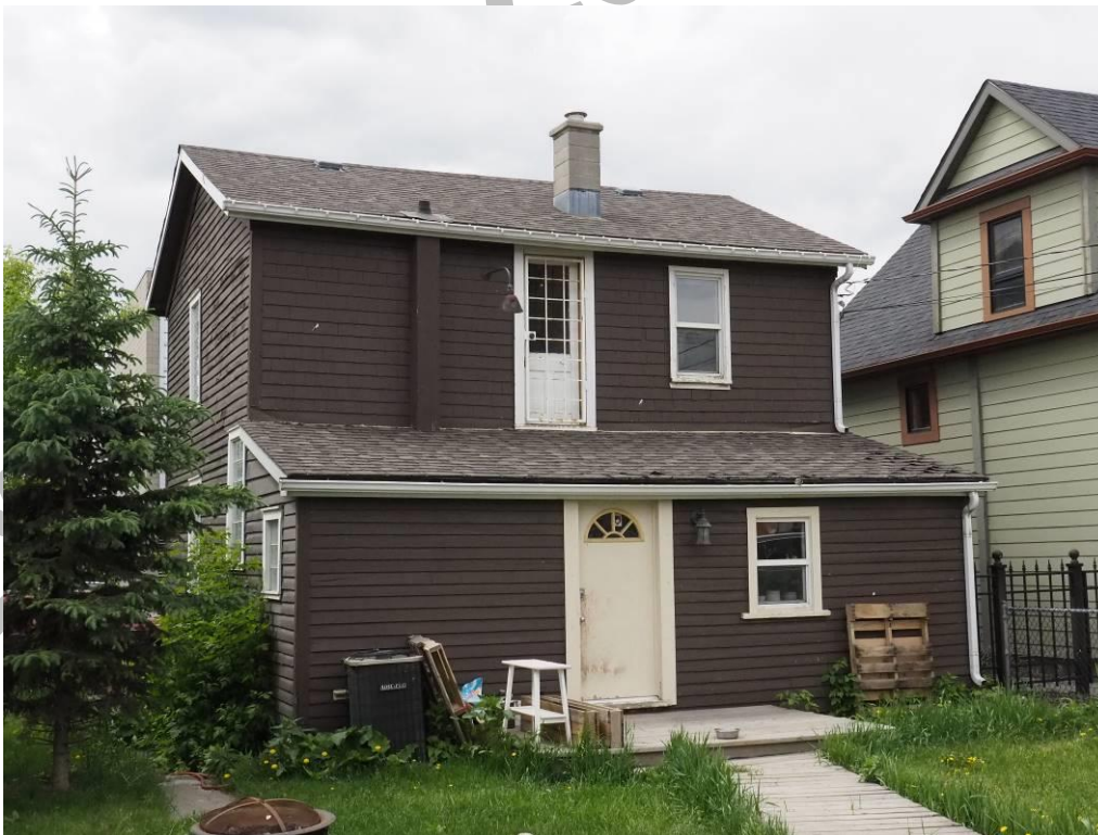
(Image 2.1 – North façade)
