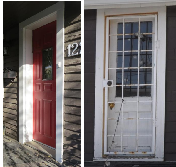
(Image 2.11 – Front (left) and second-storey rear (right) entrances)
