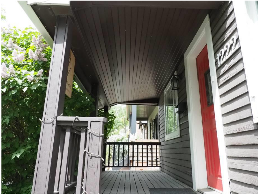
(Image 2.5 – Front verandah, looking west)
