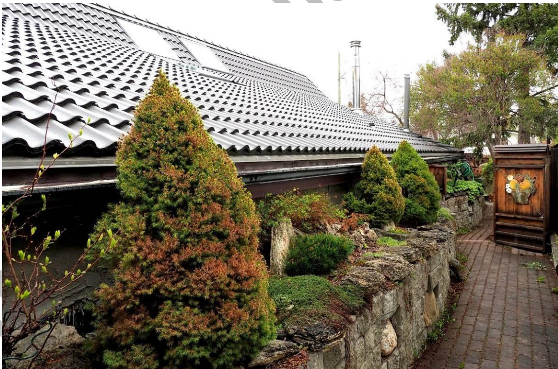
(Image 2.4 – South earth berm with 'Allan Block' retaining wall and inset local stone)
