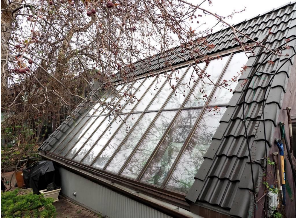
(Image 3.2 – Conservatory/garage, looking northwest)
