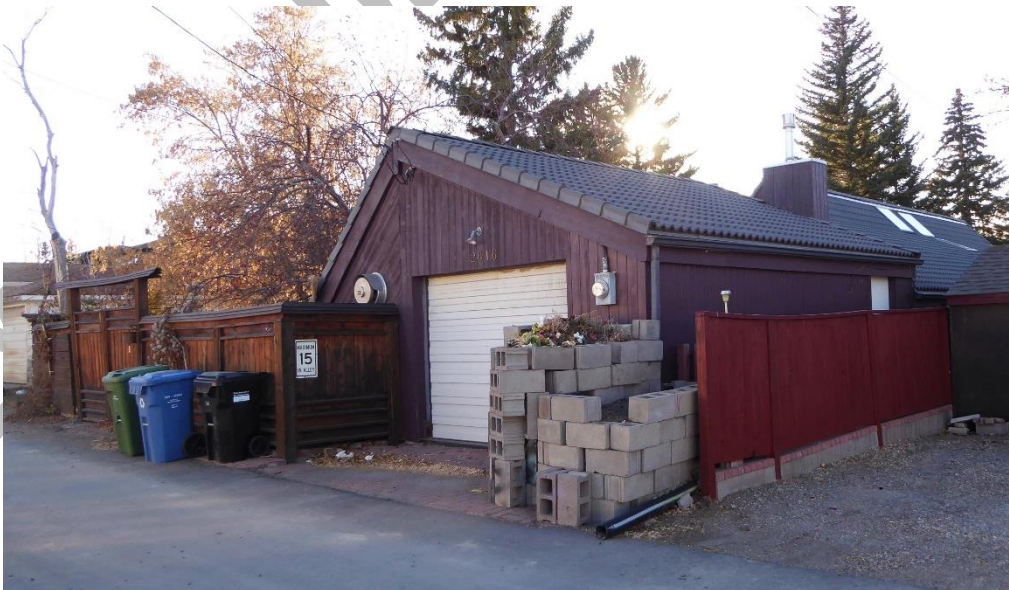
(Image 3.3 – Conservatory/garage, looking southeast)
