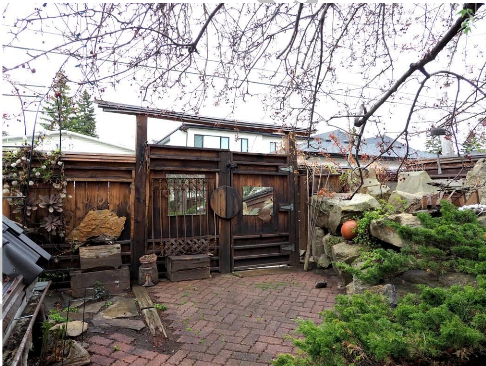
(Image 2.10 – Redwood fence and gate to alleyway; dry stacked retaining wall on right)
