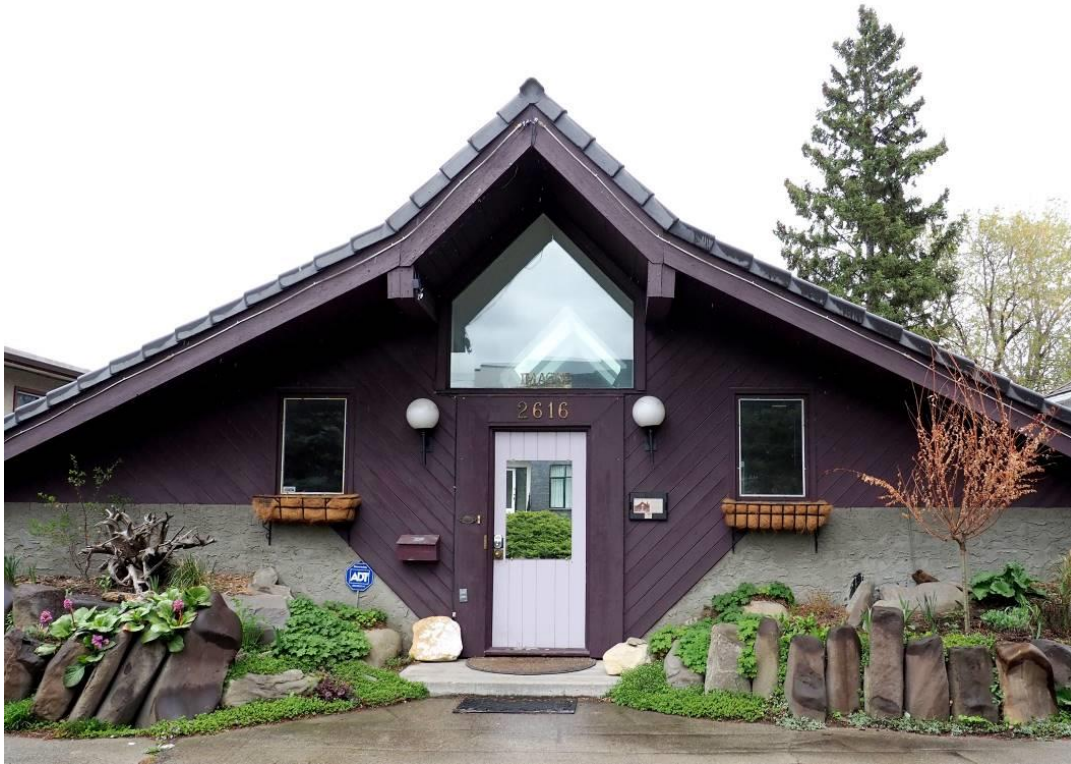
(Image 3.0 – West Façade)
