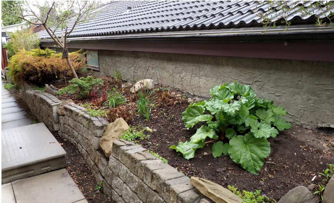
(Image 2.3 – North earth berm with 'Allan Block' retaining wall and inset local stone)
