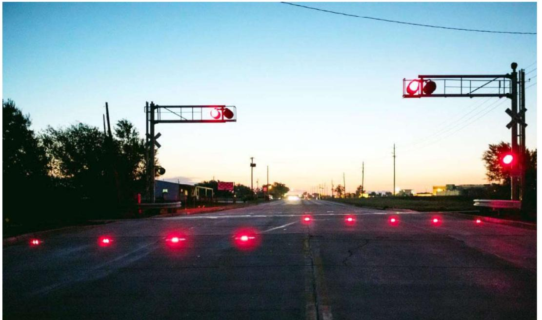
**Figure 10-3 Warning Lights Set in Pavement (LightGuard TraxAlert™)**
