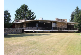
Blum Residence (built 1963) Municipal Historic Resource Designated November 2018
