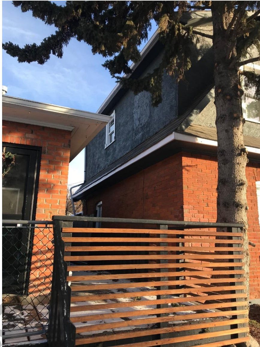
(Image 2.1: Oblique view of the north façade)
