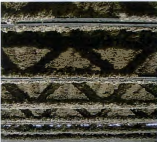
Figure C-4: Fireproofing added to structural steel
