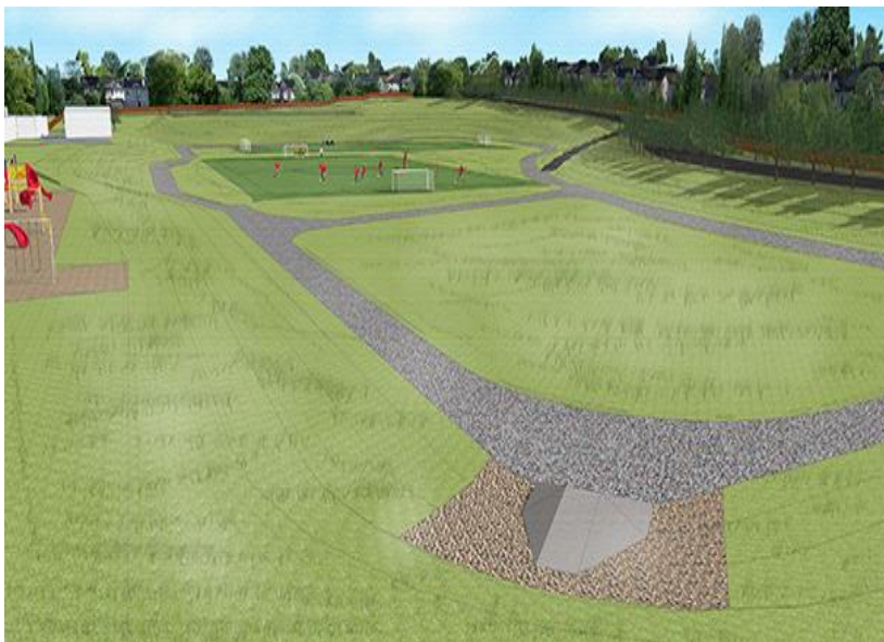
THE BRAESIDE DRY POND WILL GREATLY REDUCE FLOODING DURING EXTREME RAIN EVENTS NEAR SOUTHLAND DRIVE SW AND BRAESIDE DRIVE SW.
