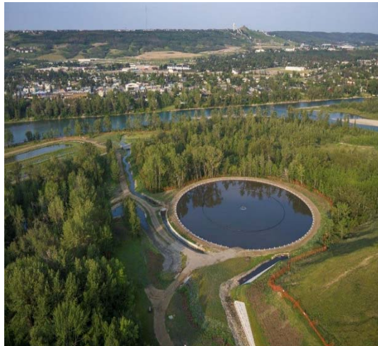
FIGURE 4.6 BOWMONT PARK - STORMWATER ENTERS THE PARK THROUGH THIS CIRCULAR NAUTILUS POND™, WHERE SEDIMENT PARTICLES ARE PREVENTED FROM ENTERING THE BOW RIVER.
