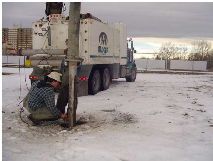
Photo 4: Hydro Vacuuming through the gravel layer (BH05)
