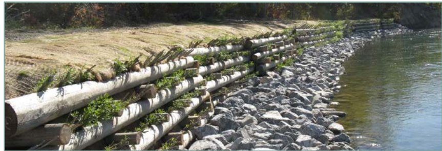
Figure 3.2 – Bioengineering Site Upstream of Glenmore Trail on Bow
