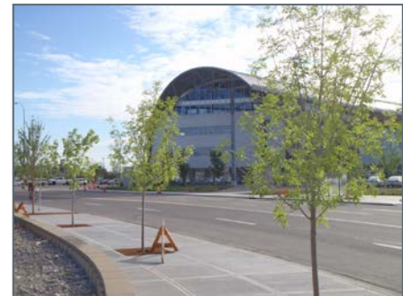
Figure 3.3 – Water Centre Soil Cell Installation
