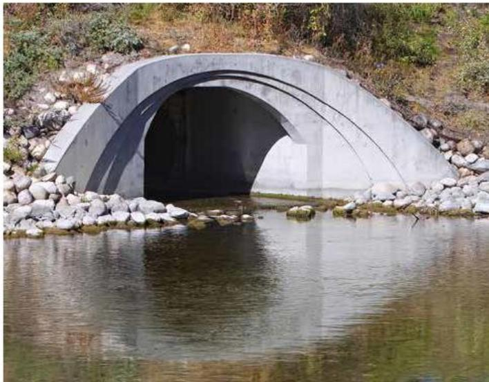
Figure 19 | Stormwater outfall
