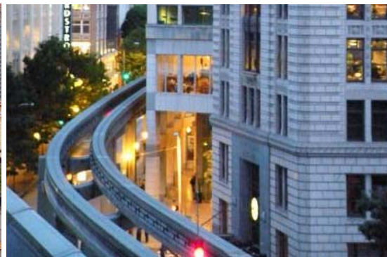
Figure 5: Westlake Tower Source: Hines
