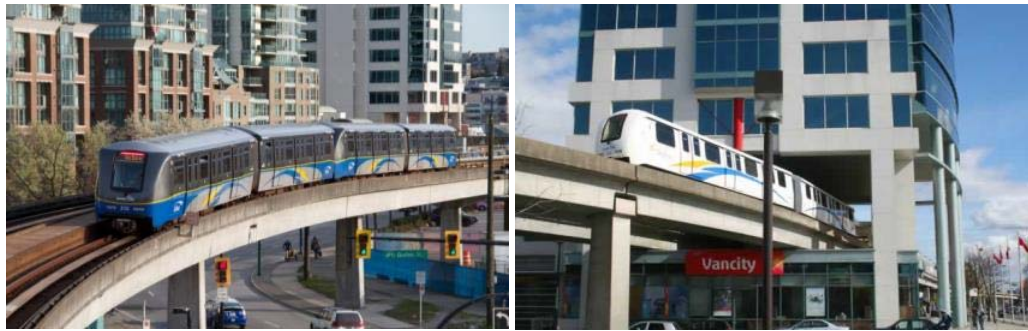
Figure 7: Vancouver SkyTrain: Terminal Avenue Source : Transport Blog
