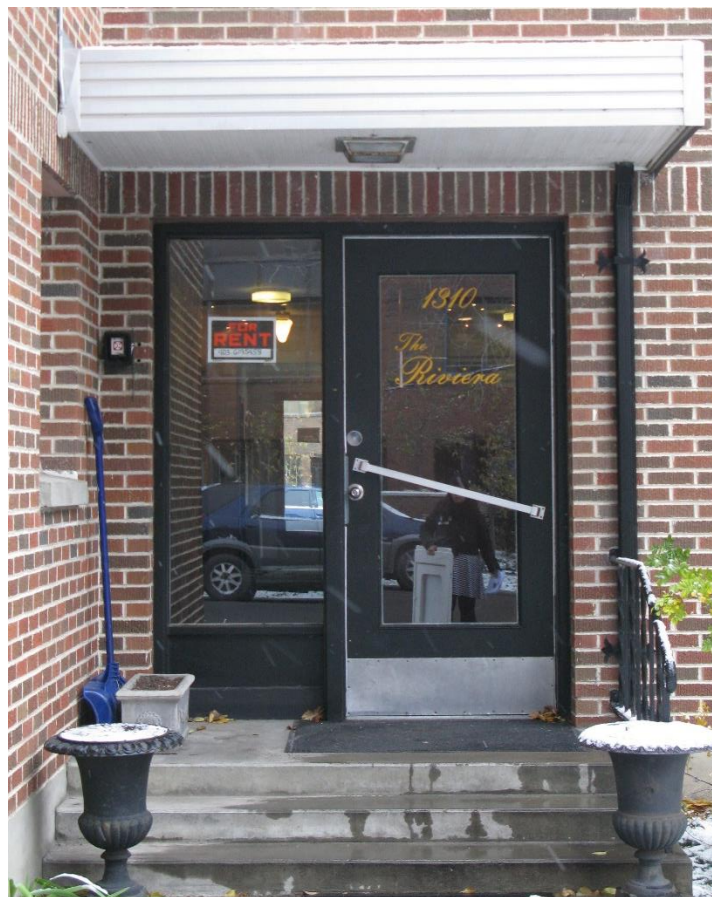
(Image 1.10: the main central entrance with wood doorway assembly, sidelight and overhang)
