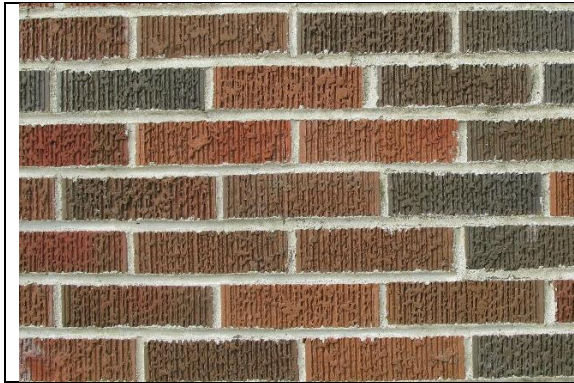
(Image 1.3: example of red/ brown vertical scored brick exterior wall in running bond)
