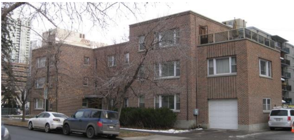
(Image 1.2: oblique view of west façade)
