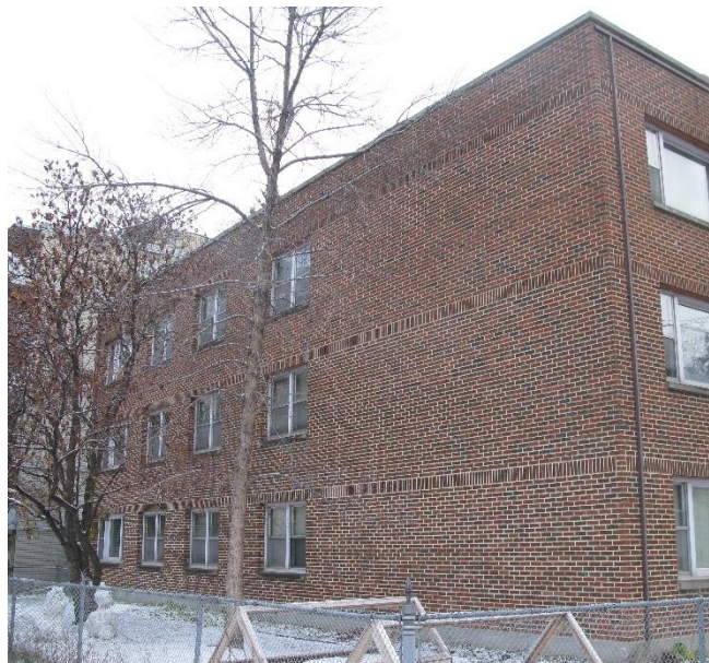
(Image 2.2: oblique view of the north façade)
