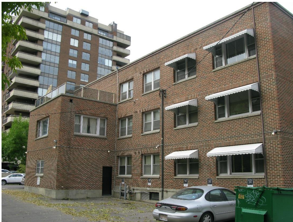
(Image 3.1: south façade)
