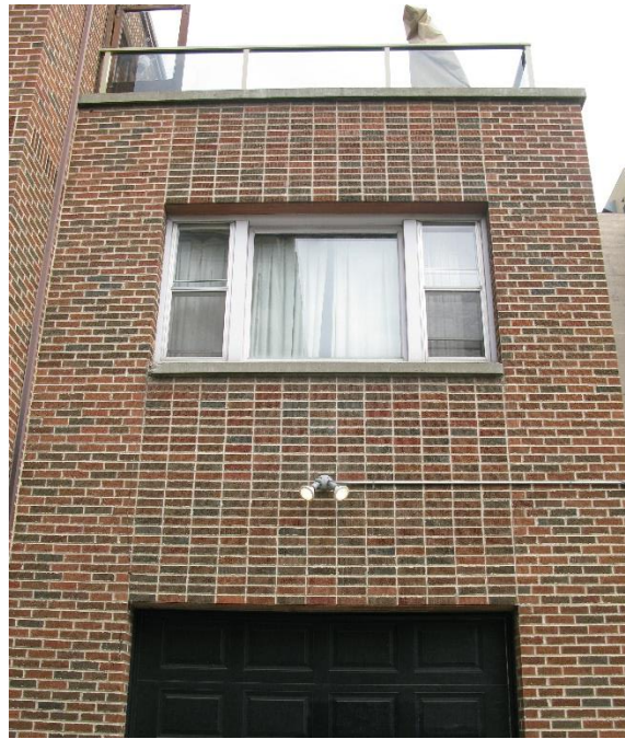
(Image 1.6: stacked bond brick detail on garage wing)
