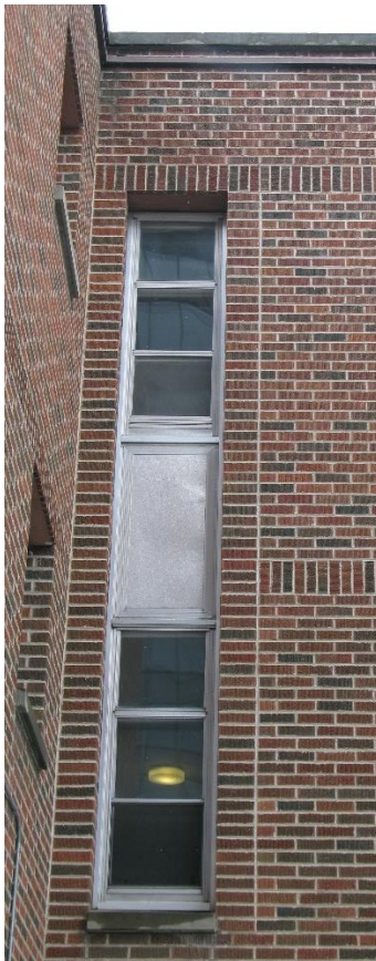
(Image 1.5: stacked bond surrounding stairwell window)
