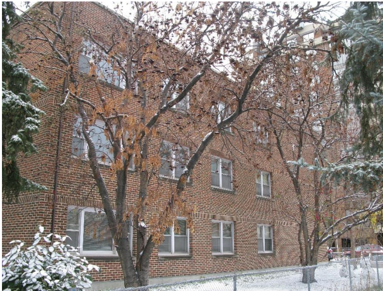
(Image 2.1: oblique view of the north façade)
