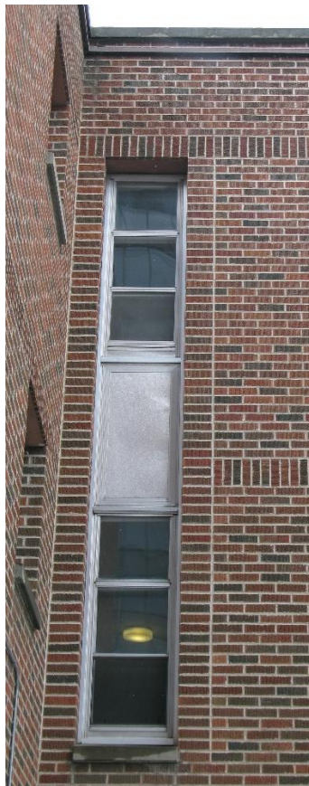
(Image 1.5: stacked bond surrounding stairwell window)
