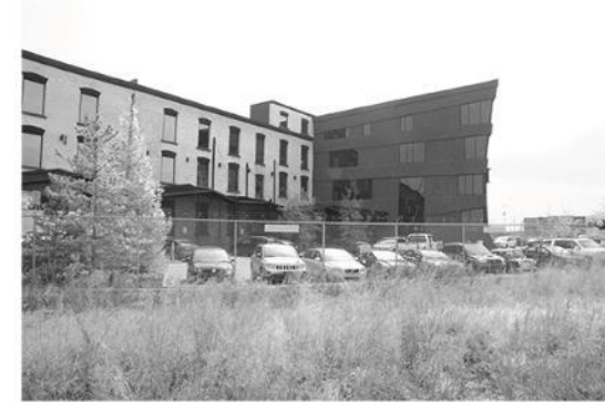
11 VIEW SOUTH EAST FROM NE CORNER OF SITE DP-0.3 / SCALE: NTS
