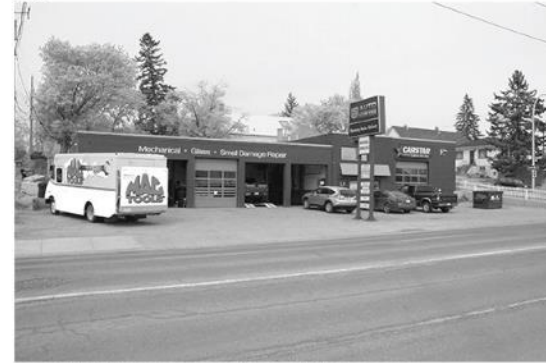
3 VIEW WEST FROM SW CORNER OF SITE DP-0.3 / SCALE: NTS
