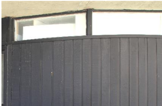
(Image 1.3: An example of the vertical board siding)
