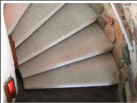
(Image 6.10: Detail of the concrete spiral cantilevered stairs, showing the treads cantilever from the outer, split faced stone clad, wall)
