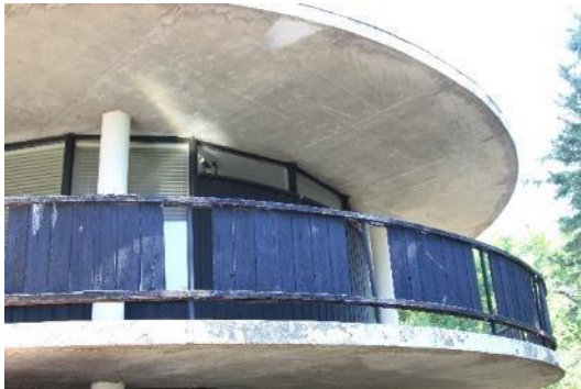
(Image 1.2: An example of the thin shell concrete roof forming the overhang and the thin shell concrete floor extending out to form the wraparound deck with continuous balustrade )
