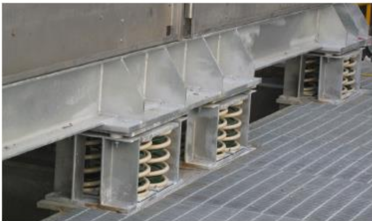
Figure 2-2: Spring Damper Isolators – Detail
