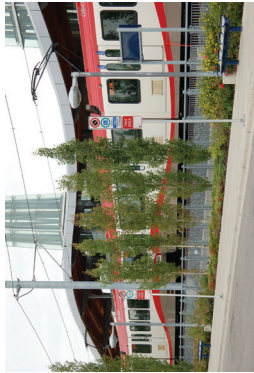
Station public realm enhancements
