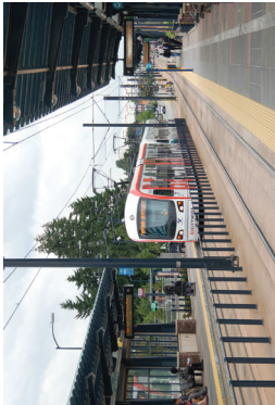
Station platforms in a low-floor system
