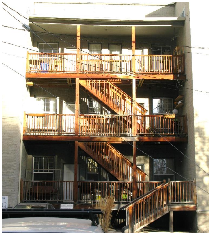
(Image 3.2: South Façade fenestration and the inset-open three storey wooden porch with stairs from grade to third floor)
