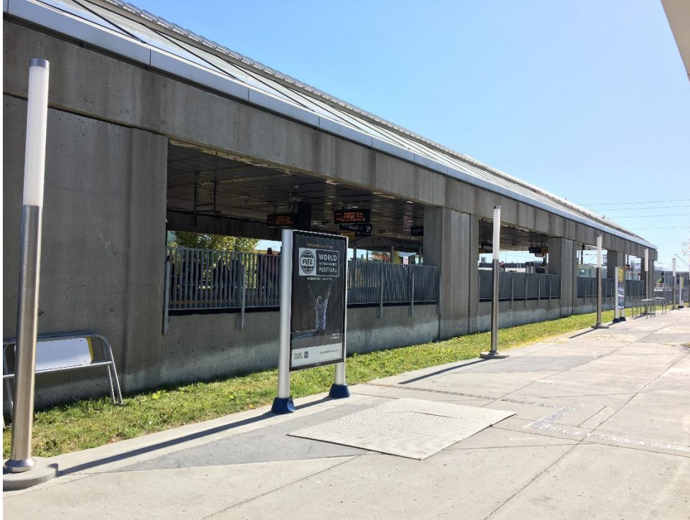
View looking south at Chinook LRT Station signage. Sign is two metres high.
