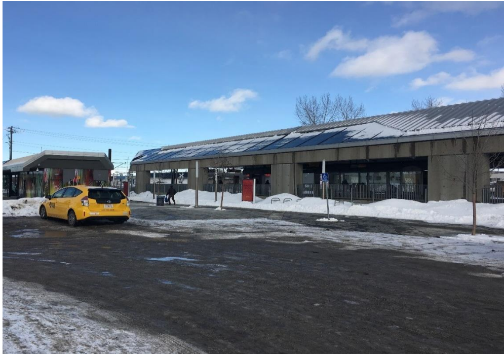
View looking northeast at Chinook LRT Station
