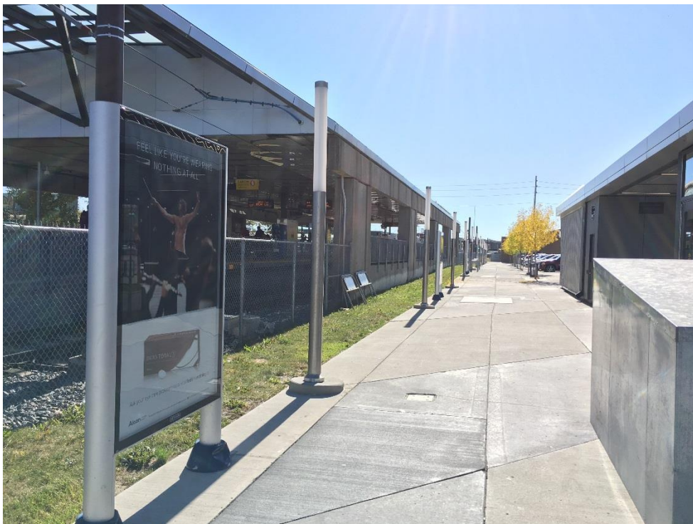
View looking south at Chinook LRT Station signage. Signs are approximately 20 metres apart.
