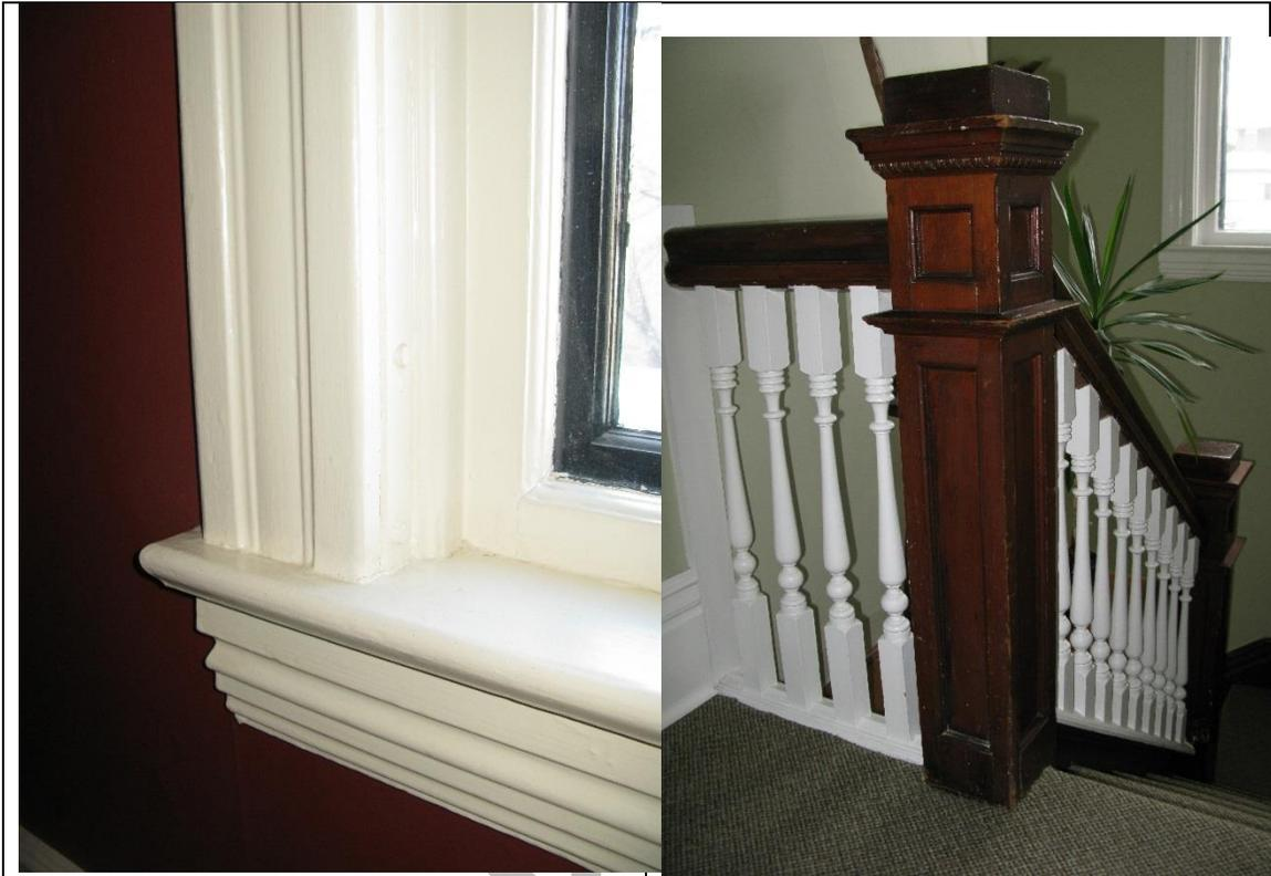
Image #6.2 – Example of a portion of the window casings used throughout the house
