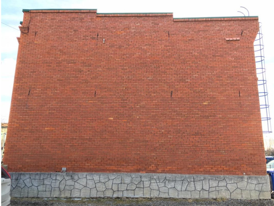
(Image 2.1: North Façade)
