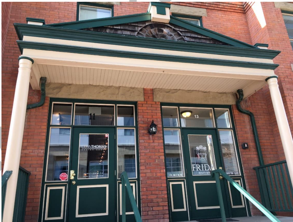
(Image 1.3: Detail view of an East Façade porch and replacement doorway assemblies)
