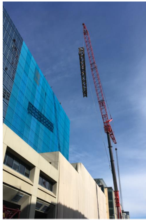
Box Truss Installation
