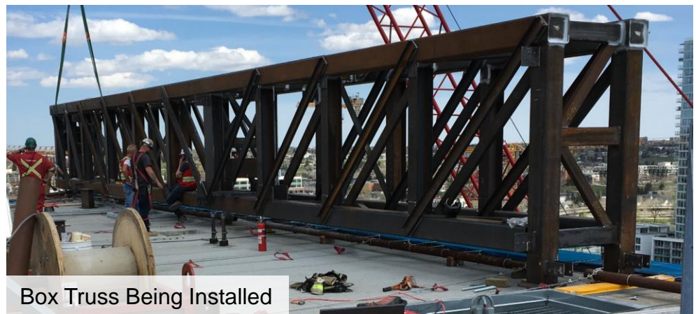
Box Truss Installation
