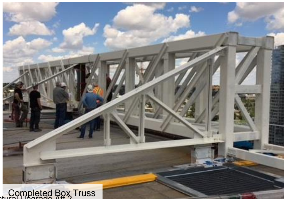
Box Truss Being Installed
