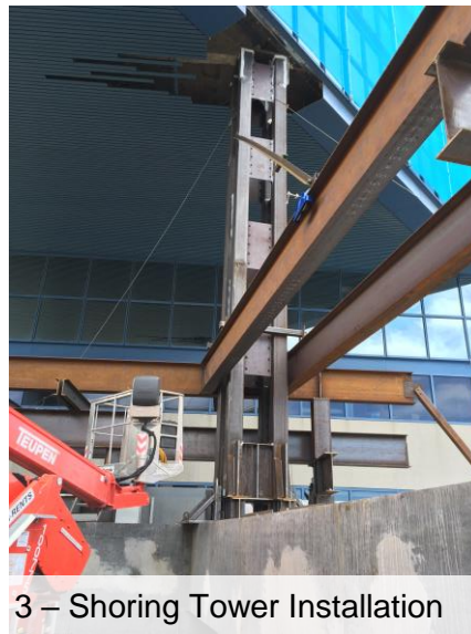
2 - Shoring Tower Installation
