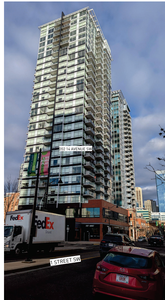
9 EXISTING SITE PHOTO FACING NORTH WEST N/A
