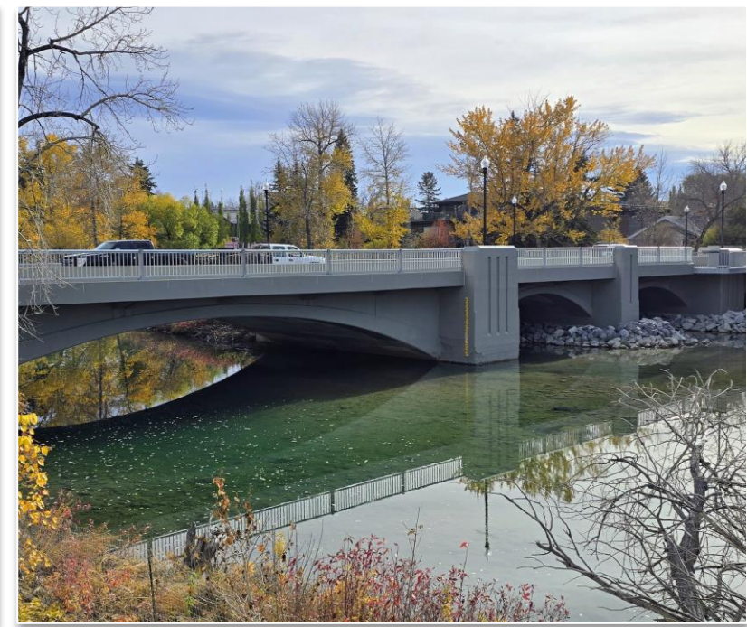
Mission Bridge Rehabilitation
