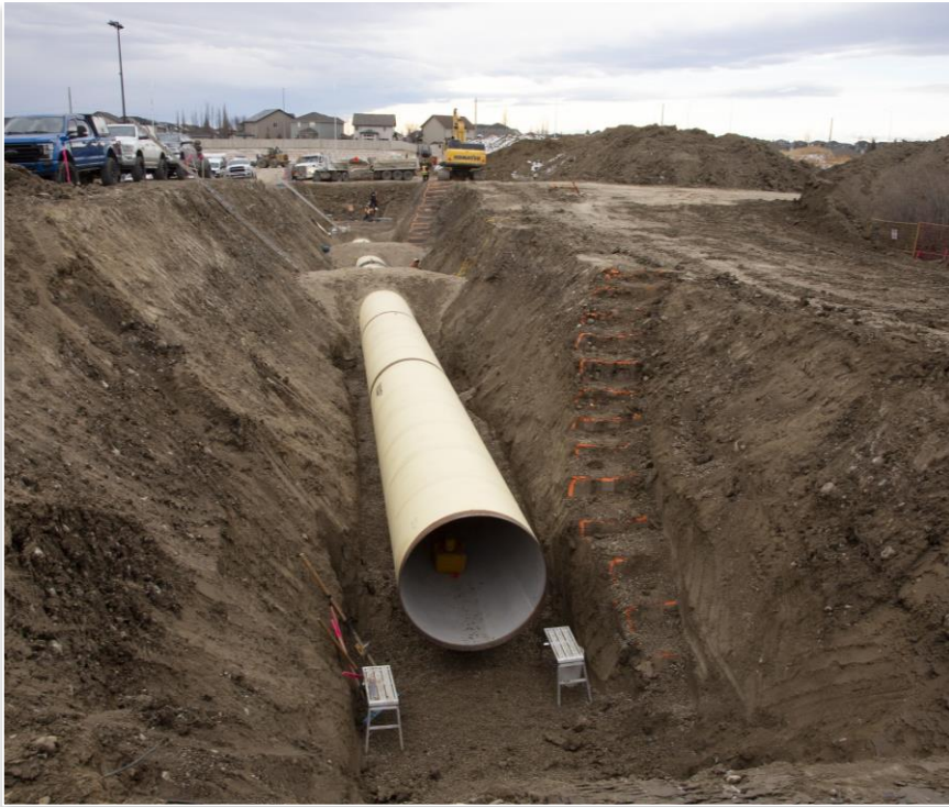
North Calgary Water Servicing
