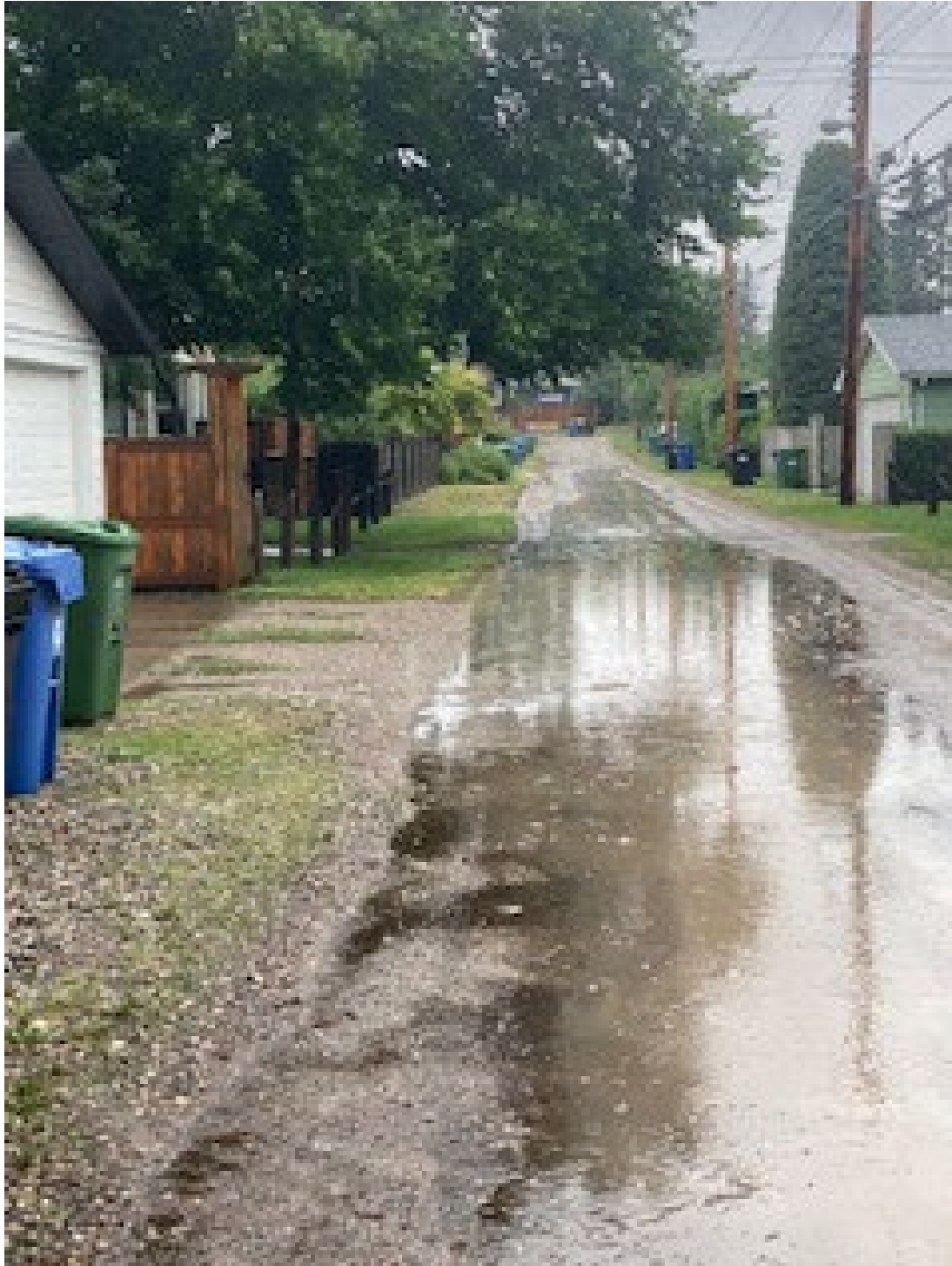
Exhibit 2 – Lane Way Water (reaching limits of containment)
