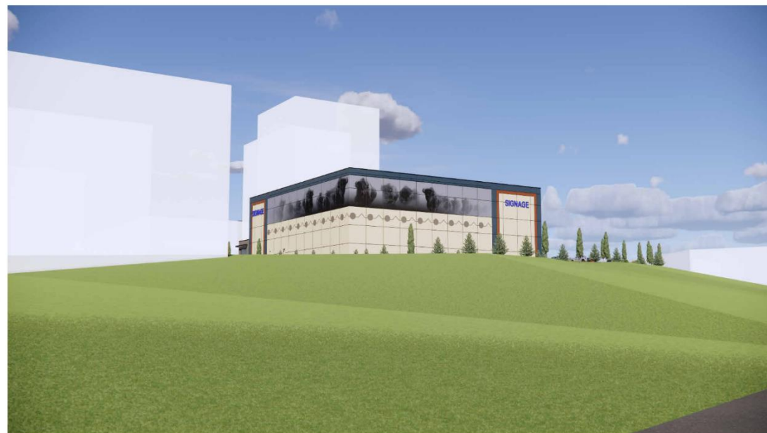
VISUAL IMPACT - TRANS CANADA HIGHWAY (DISTANCE OF 150m)
