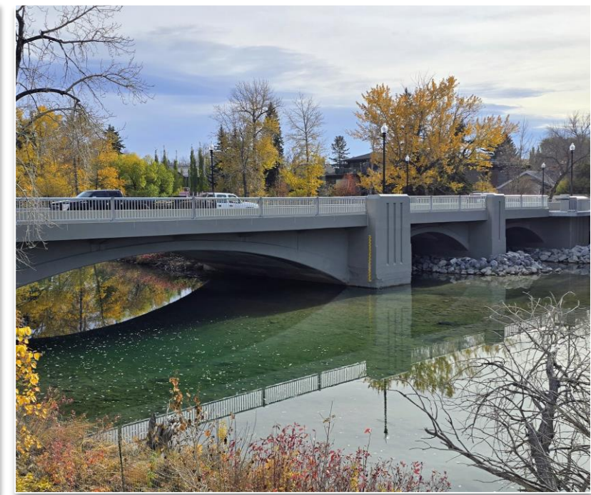
Mission Bridge Rehabilitation
