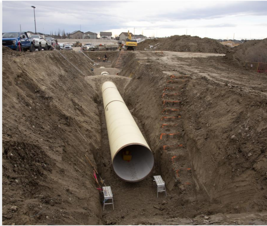
North Calgary Water Servicing
