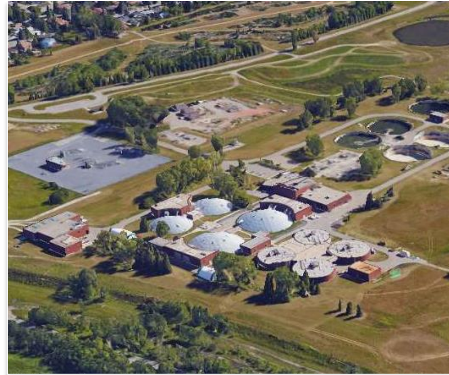
Fish Creek Wastewater Treatment Plant Upgrades
