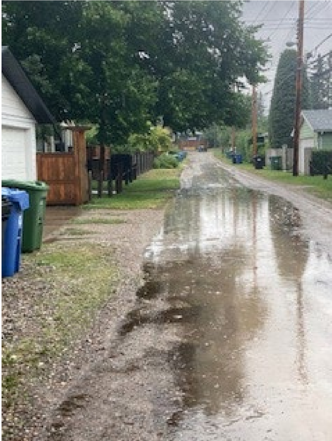
Exhibit 2 – Lane Way Water (reaching limits of containment)
