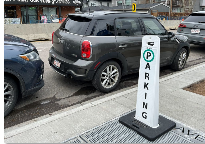
Construction Area Parking Management (on-street parking)
