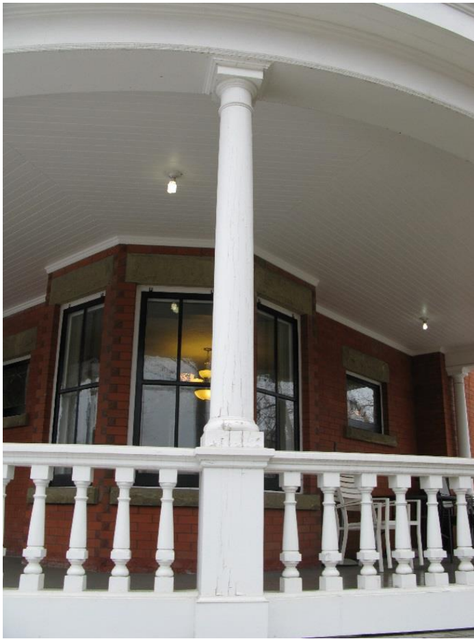
(Image #1.6 – Detail view of the veranda, showing balustrade, Tuscan-style column and wooden tongue-and-groove ceiling)
