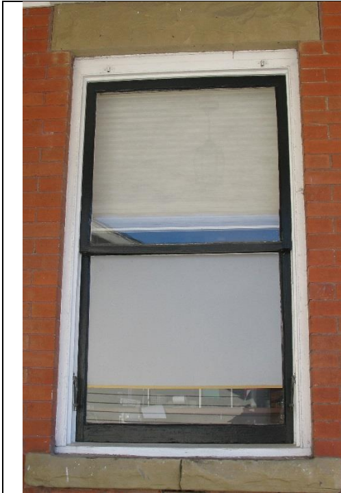
(Image #1.3 – Example of a 1-over-1 wooden-sash window common to all façades; sandstone lintel above the window opening and sill below)
