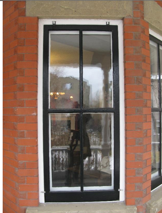
(Image #1.4 – Example of a window with 4-pane wooden storm sash)
