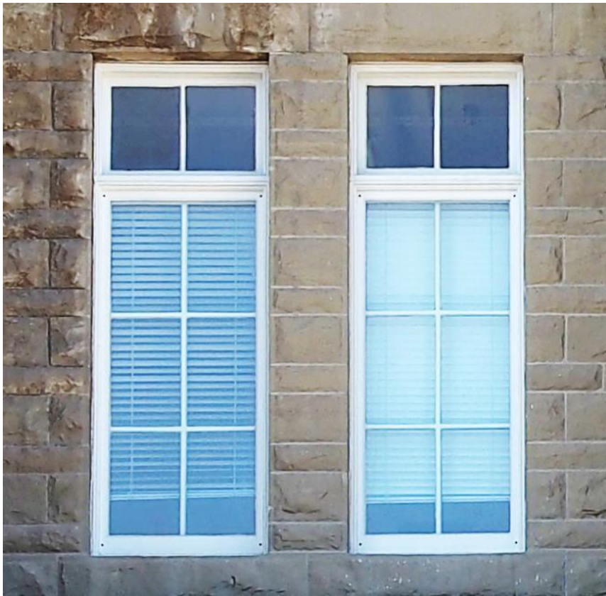
(Photo 1.5: An example of the wooden-sash, six-pane windows with two-pane transom lights)
