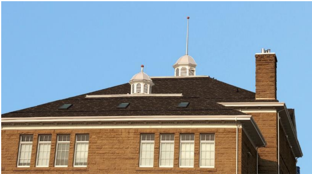
(Photo 5.1: Roof elements – detail view showing the two extant cupolas)
