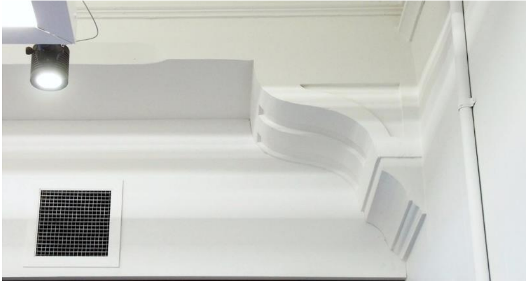
(Photo 6.1.05: First Floor – former auditorium space showing plaster ceiling beams and decorative brackets)
