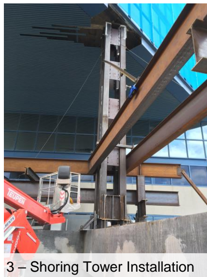
2 - Shoring Tower Installation
