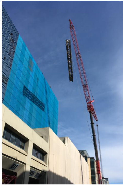
Box Truss Installation
