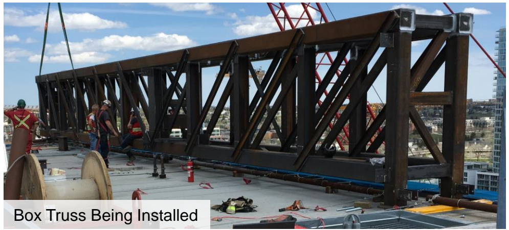
Box Truss Installation
