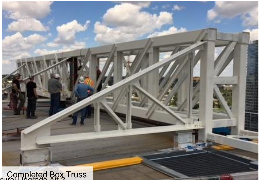
Box Truss Being Installed
