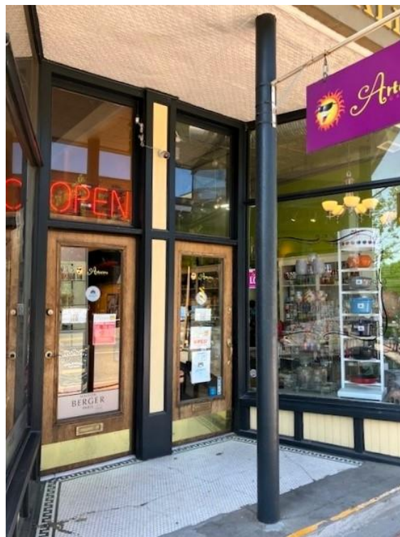
(Image 3.12: Example of recessed entry and steel column)
