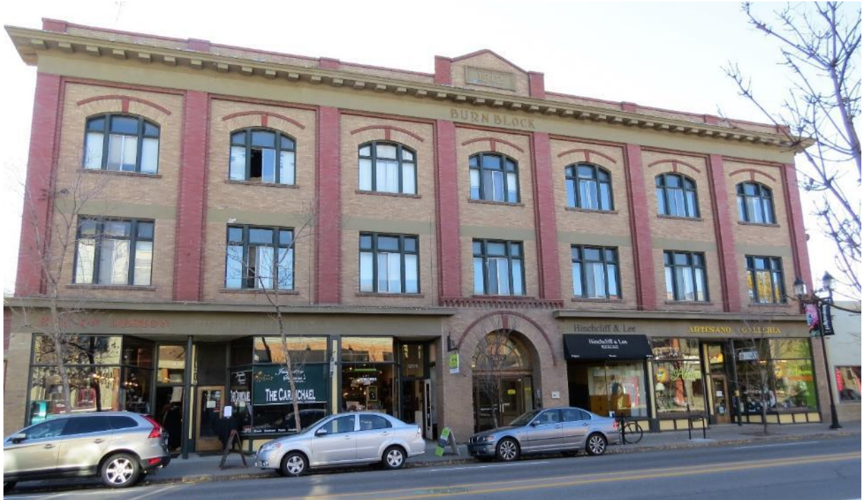
(Image 3.1: North façade showing three storey, rectangular plan, polychrome brick cladding, pedimented stepped gable and red-coloured brick pilasters framing window grouping bays)
