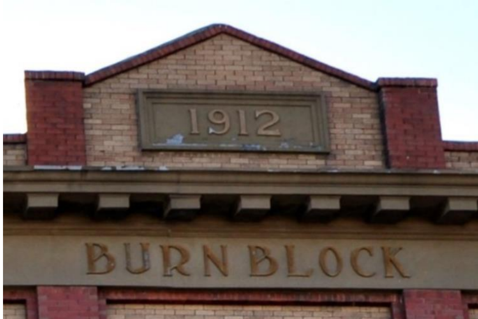
(Image 3.4: Detail of buff-coloured brick pedimented stepped gable with red-coloured brick coping at the roof edge and '1912' numbering)
