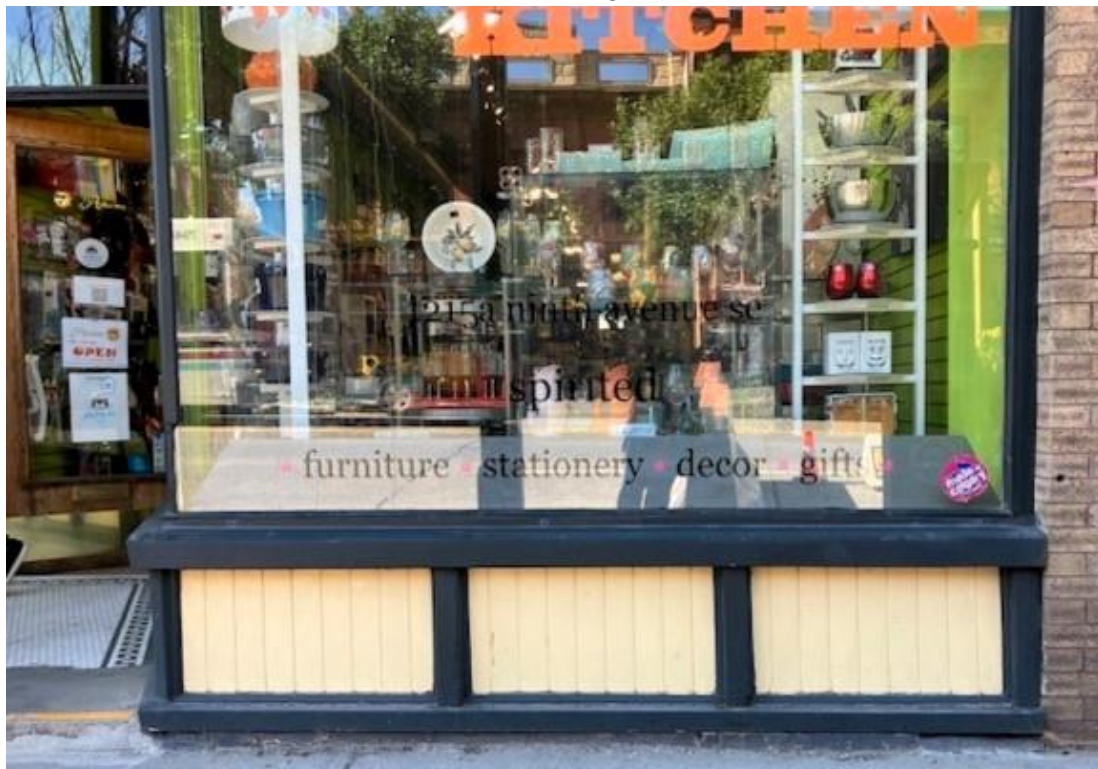
(Image 3.9: Example of wood panel bulkheads)
