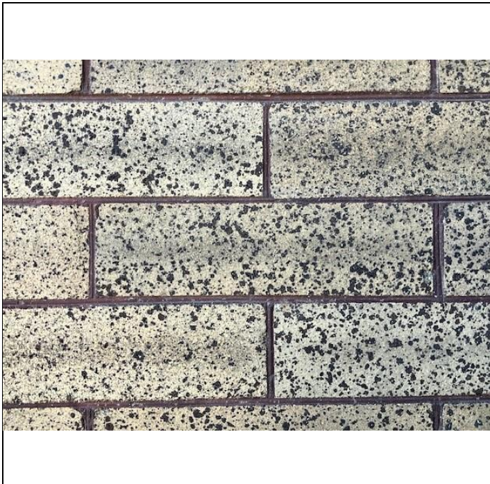
Image 3.2: Detail of buff coloured speckled brick cladding in stretcher bond pattern with beaded joint on north facade.
