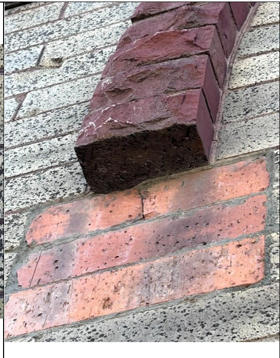
Image 3.3: Example of polychrome brick cladding showing buff-, light red-, and red-coloured bricks.
