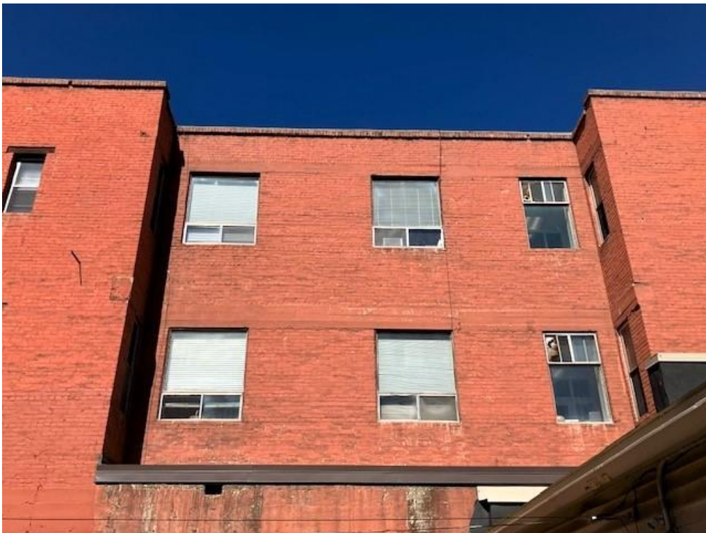
(Image 4.3: Detail of light well on east façade)
