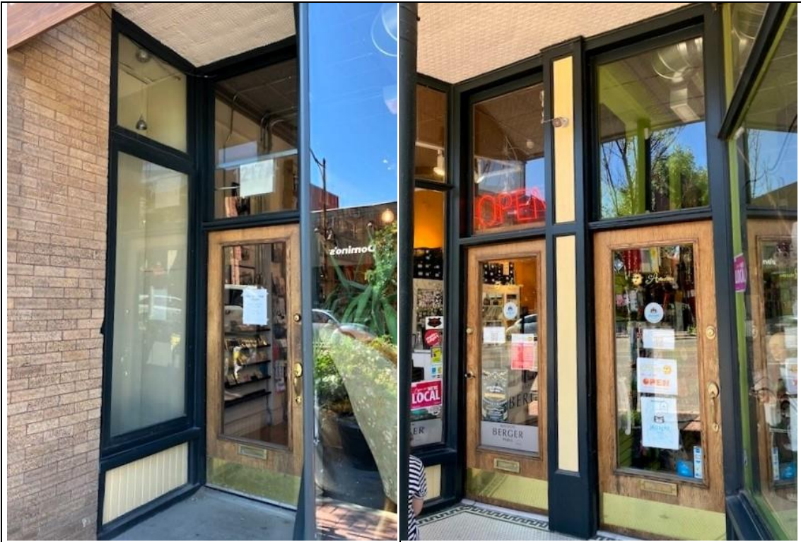
Image 3.10: Example of glazed display case in west side of central main entry.
