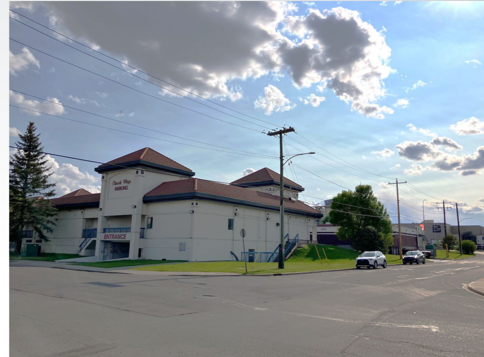
Site from the northeast; 60 Avenue SW and 3 Street SW
