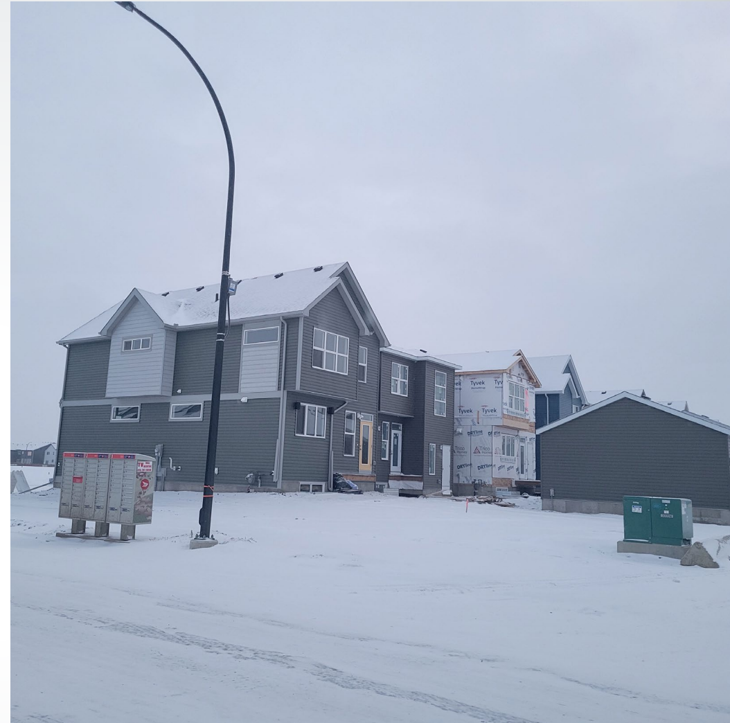
Site from northeast corner (near junction 45 ST SE & rear lane )
