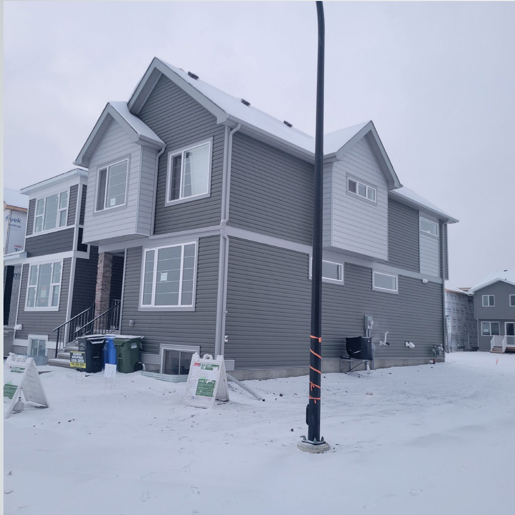
Site from southeast corner (near junction Setonstone GR SE & 45 ST SE )
