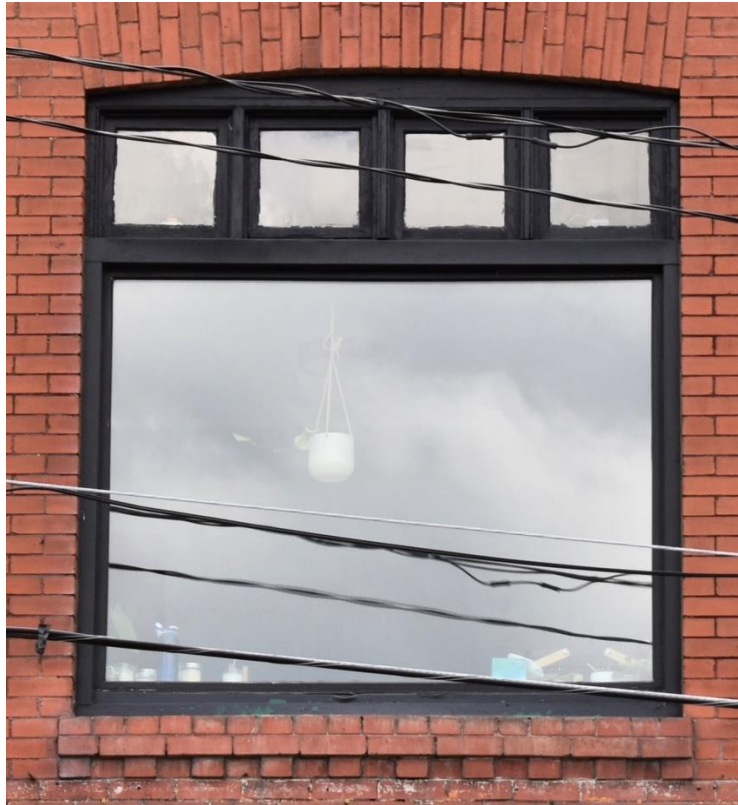
(Image 1.1: Example of an upper storey window and wood sashes)
