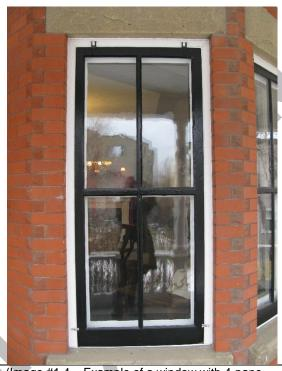
(Image #1.4 – Example of a window with 4-pane wooden storm sash)
