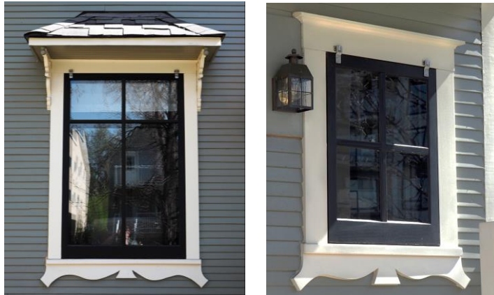
(Image 2.9: Detail of main floor regulated windows on north façade, showing restored original wood sash windows and reconstructed wood storm sashes)
