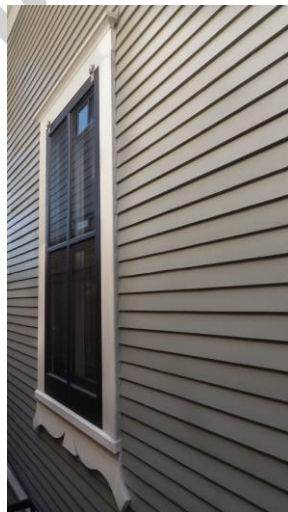
(Image 2.11: Detail of regulated window on east façade, showing restored original wood sash window and reconstructed wood storm sash)
