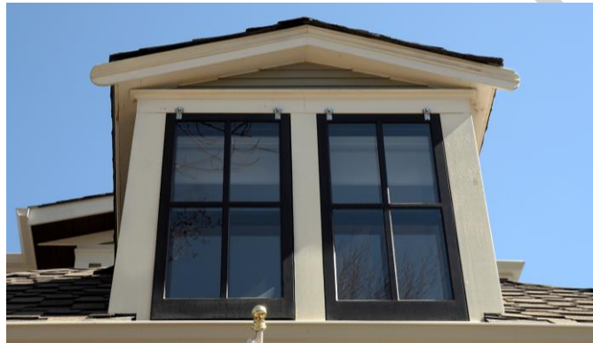
(Image 2.10: Detail of second-storey dormer on north façade, showing restored original wood sash windows and reconstructed wood storm sashes)
