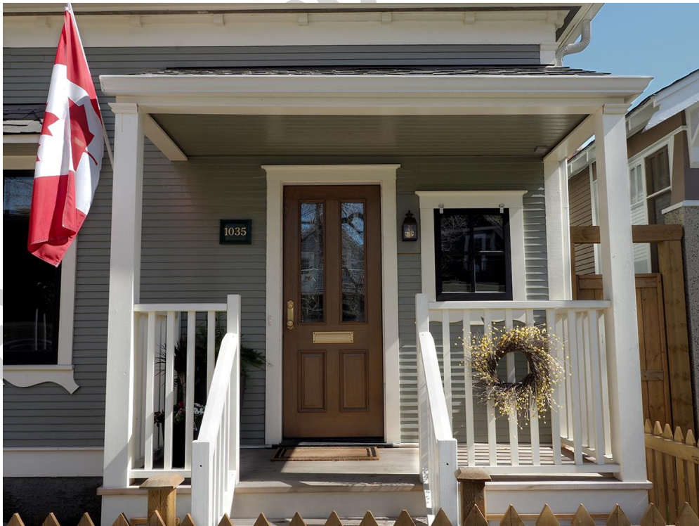
(Image 2.8: Reconstructed front porch on the north façade, including restored shed roof; existing platform, supports and balustrade are not regulated)
