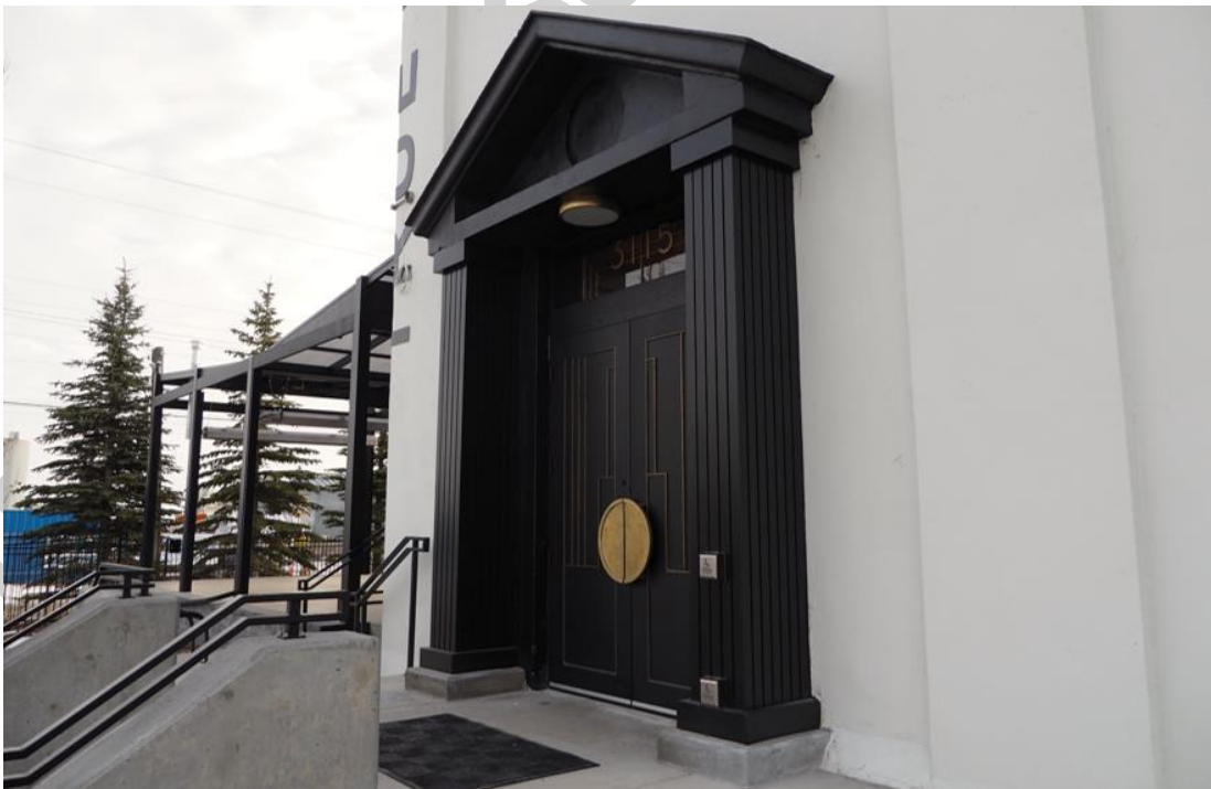
(Image 3.11: Detail photo showing profile of regulated cast concrete pediment; columns below pediment and doors are not regulated)
