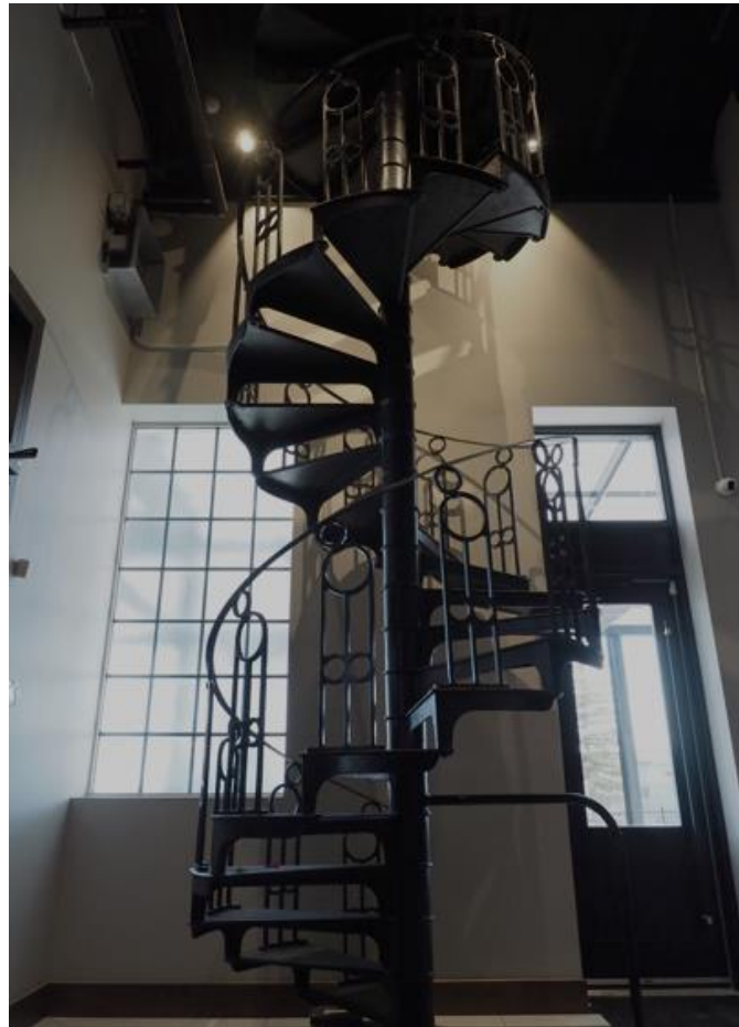
(Image 4.0 – Interior photo showing regulated metal spiral staircase; staircase currently capped and top of center column removed)
