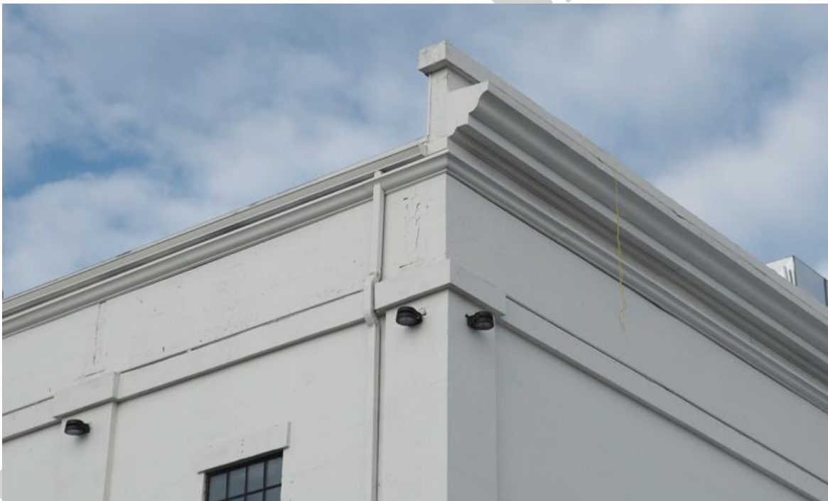
(Image 3.9: Detail photo showing profile of parapet, eave-height cornice, and flat-roof)
