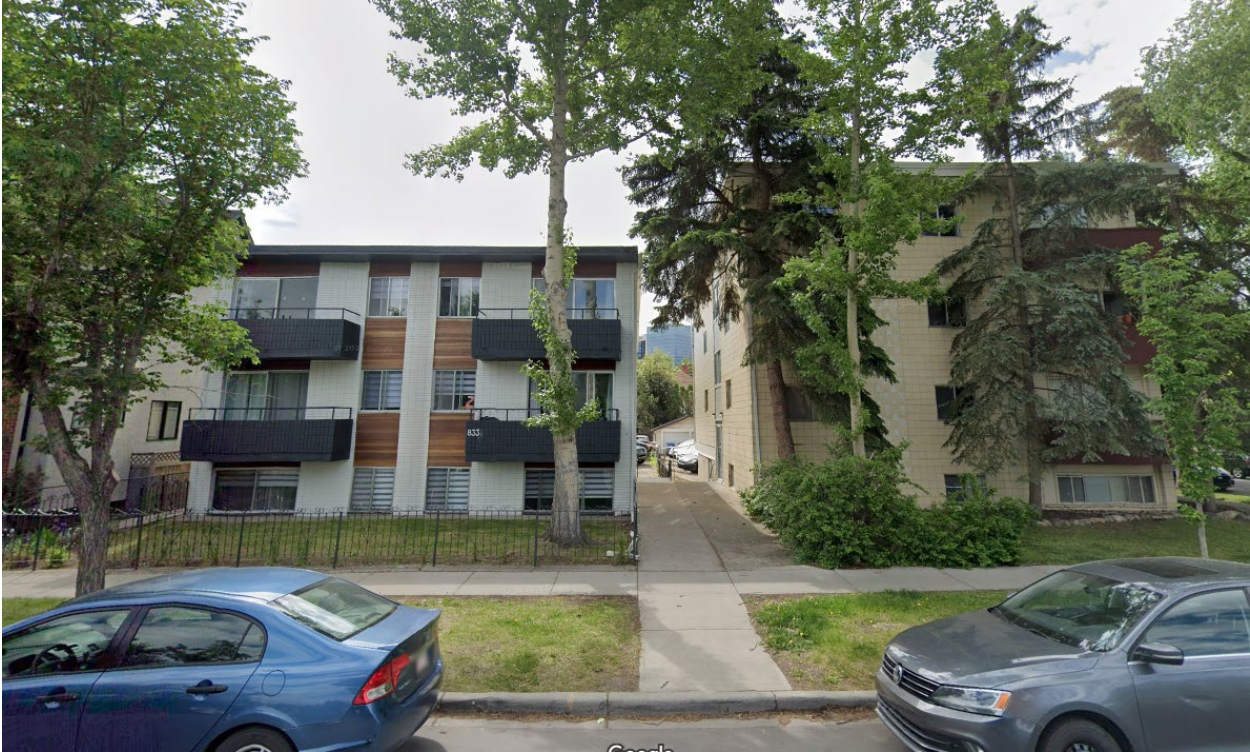
Apartment buildings at the west end of the 800 block
