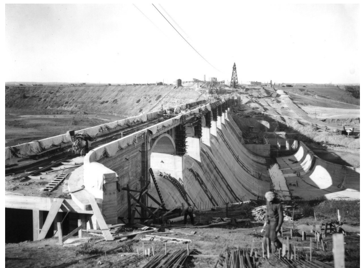
View of the Glenmore Dam nearing completion, 1931. Glenbow Library and Archives Collection, Libraries and Cultural Resources Digital Collections, University of Calgary
