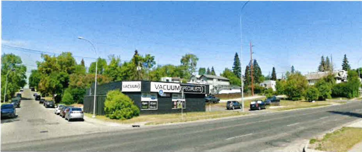
SE Corner – one building located on the southern parcel looking NW from Centre St N and 30 Avenue NE
