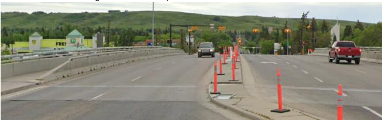
Photo 2: The set of traffic lights at Charleswood / 32 nd
