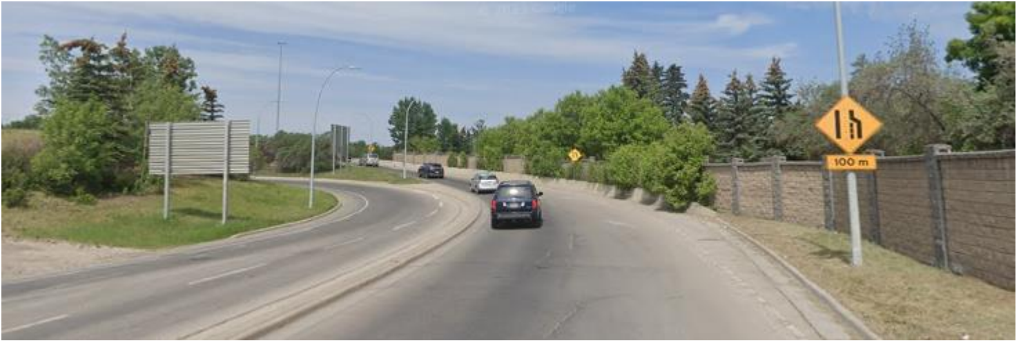
Photo 10 – Access ramp onto Crowchild Trail North
