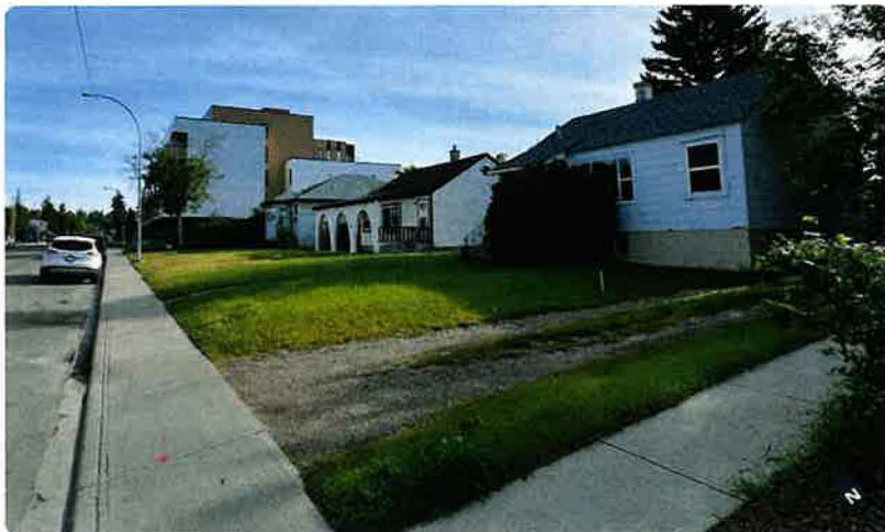
19 ST NW looking North
