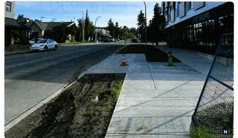
19 ST NW looking North
