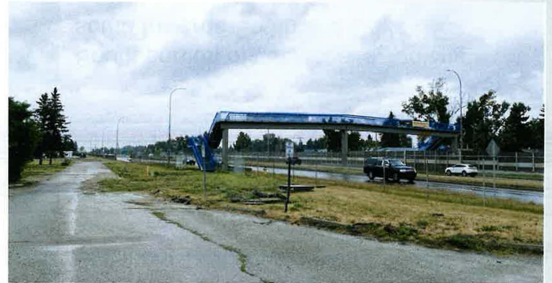
Existing Pedestrian Bridge over Blackfoot Trail.
