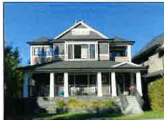
Recessed upper deck
