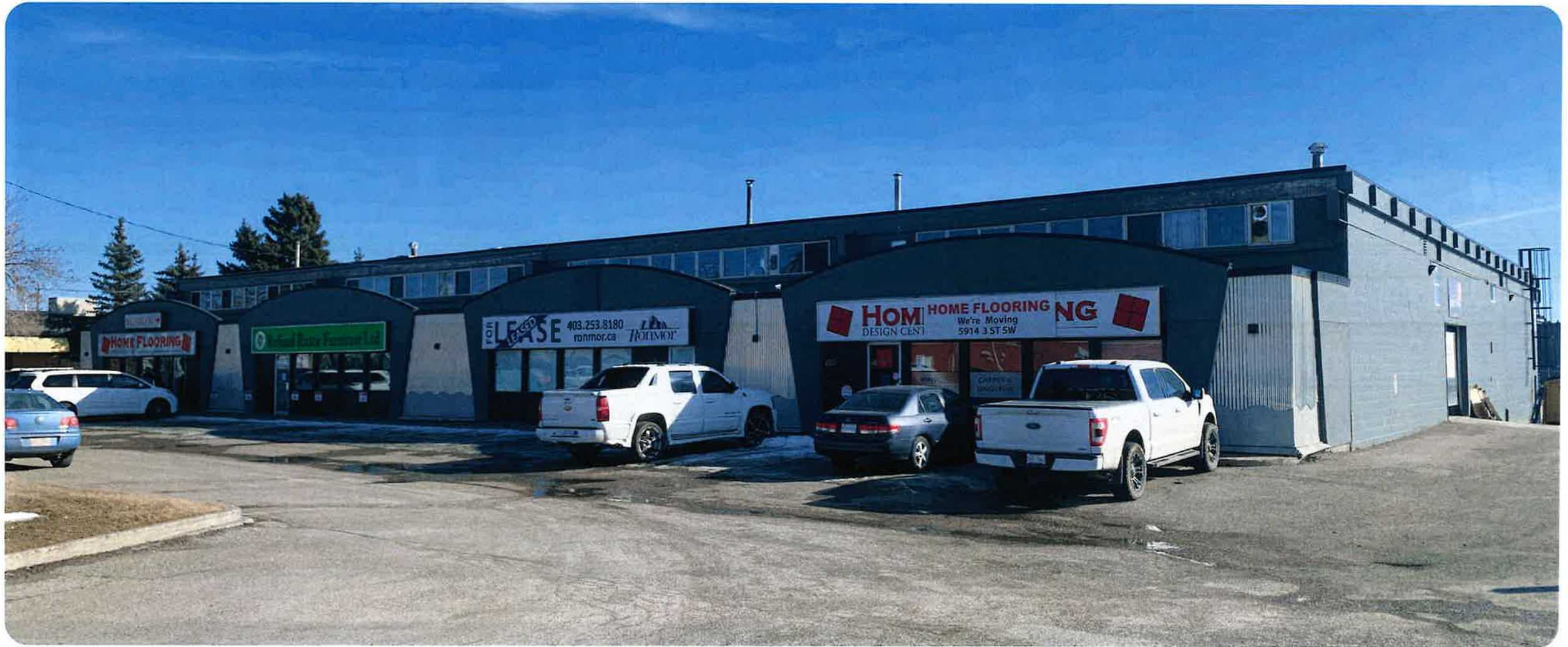
Subject Site (View southeast towards existing building)
